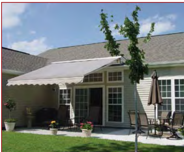
Roof Mount installation
